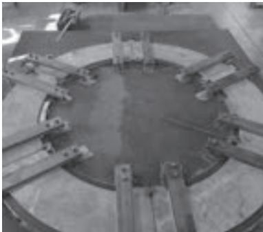
Welding using Fixtures
