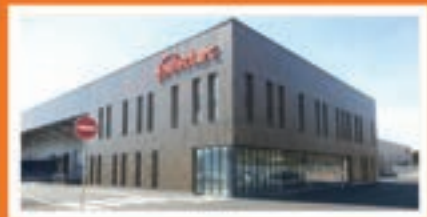
New plant at Grandvillars-France
