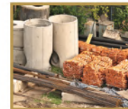
Building Material Testing
